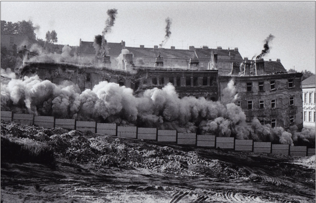
Iren Stehli, demolition of buildings at Komenského square, circa 1980
