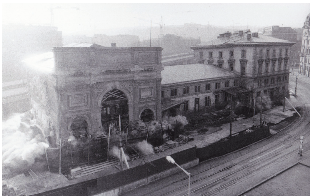
Demolition of the Praha-Těšnov train station by Carl Schlimp, 1872–1875. Photo ČTK, 1985
